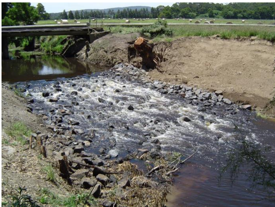
Figur 6. Gellibrand rock ramp fishway (Photo Steve Saddlier).
